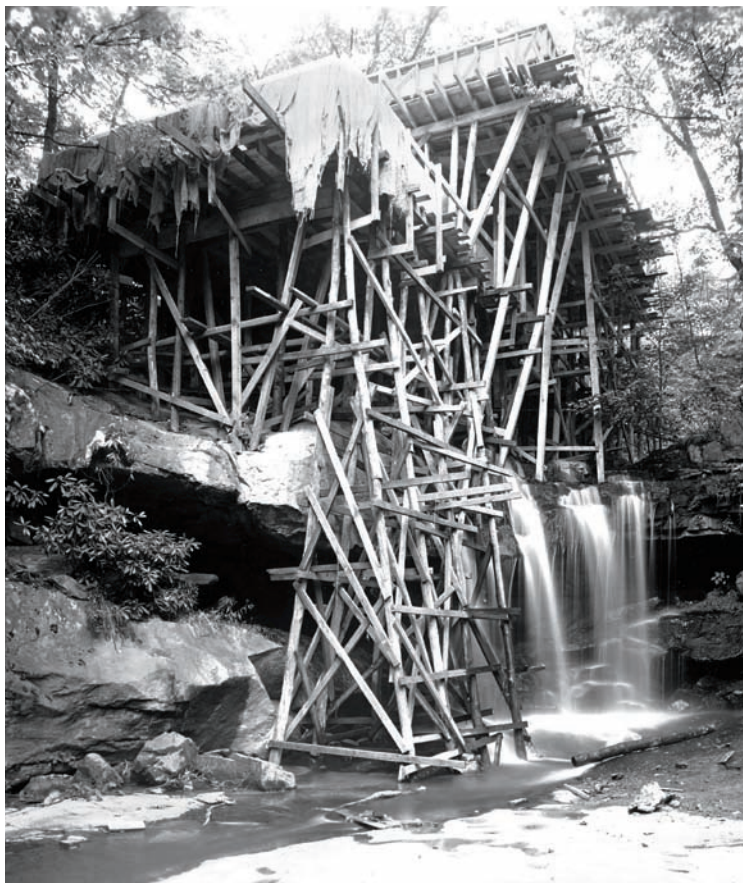
Construction of Wright's Fallingwater
